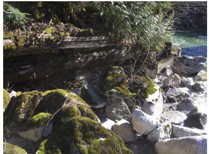
Upstream right bank
