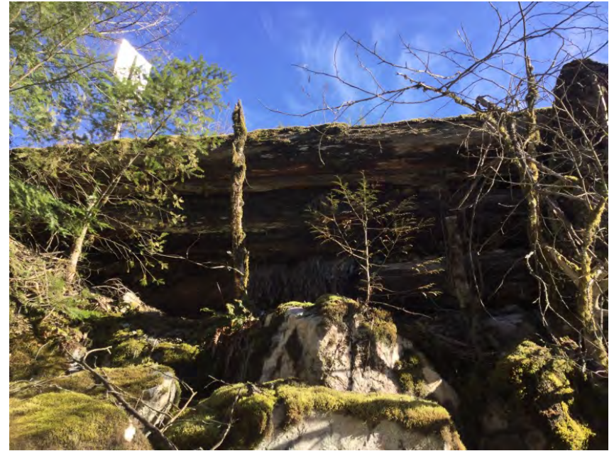
Wingwall upstream left bank
