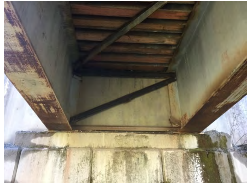
New end diaphragm at right abutment
