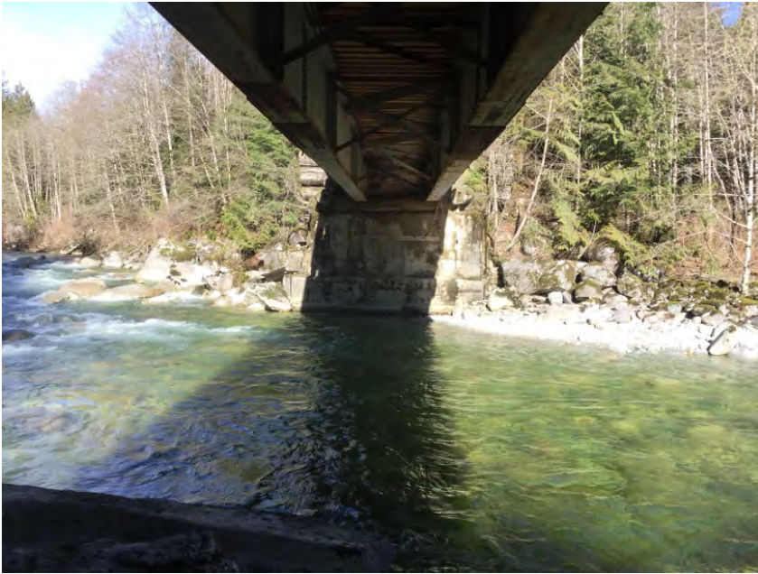
Left Bank Abutment when facing downstream
