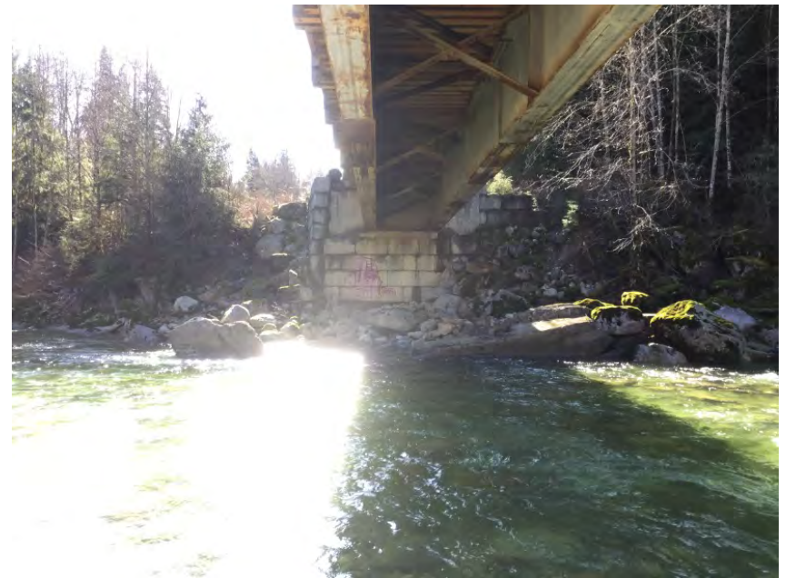
Right Bank Abutment when facing downstream
