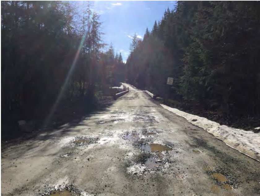
Approach from Left Bank when facing downstream
