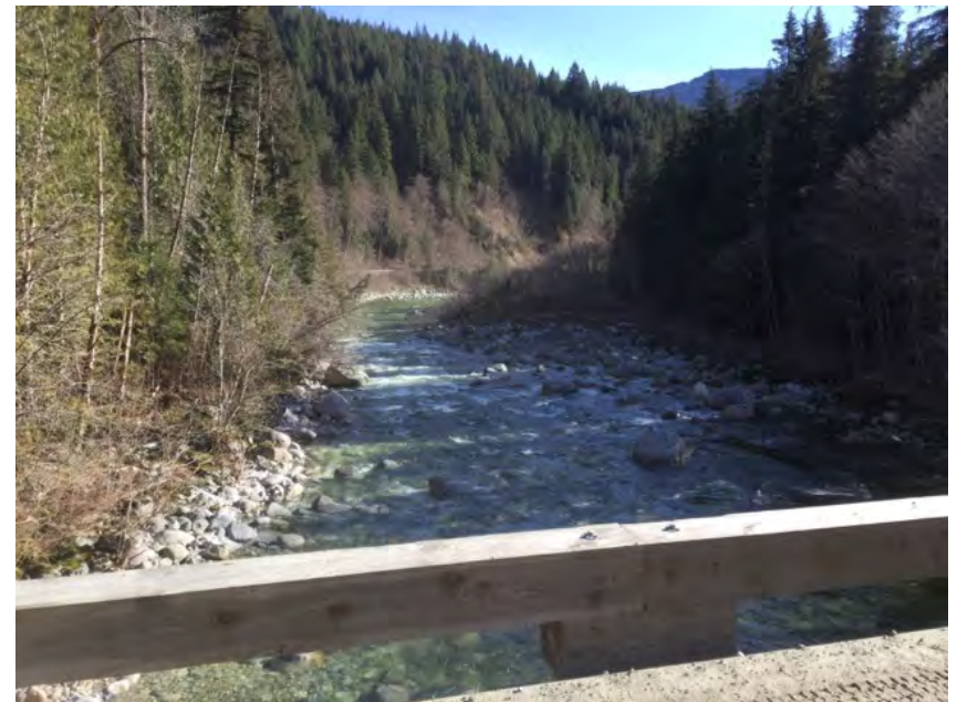
Looking downstream from deck
