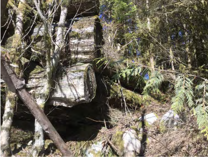
Downstream left wingwall
