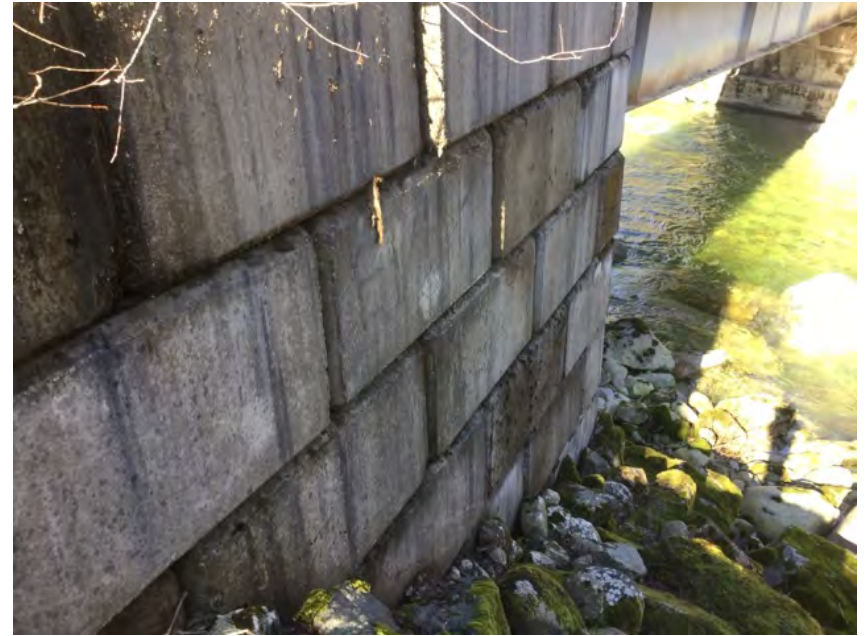
Lock block wingwall at DS right abutment
