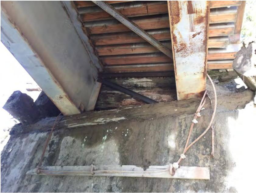
New end diaphragm at left abutment
